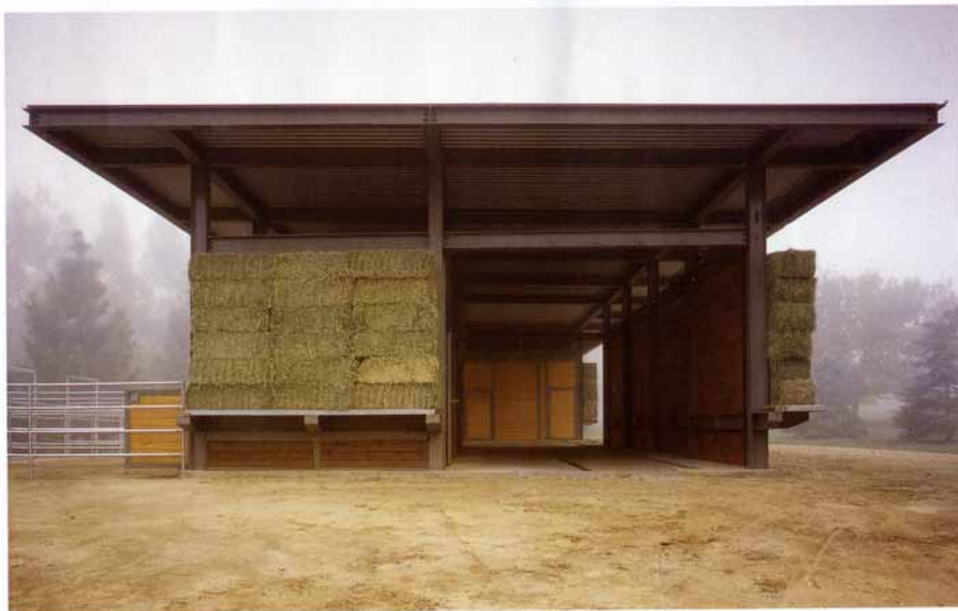
The metal roof deck extends well beyond the barn's edges to protect interior spaces and the stacked bales of hay from the rain.
