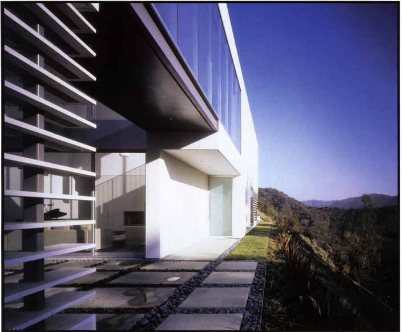
Louvers on the east façade of the Bel Air residence are made of limestone. Architect Zoltan Pali told the contractor, who had never before installed stone louvers, to “think of them as a bunch of countertops” (facing page and above). The glass-enclosed second-story bridge takes advantage of expansive, downhill views (below).
