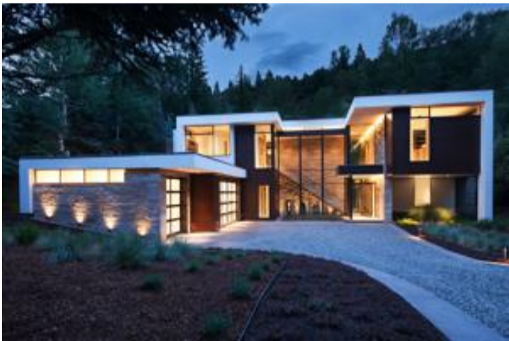
08-.3980 Fourteen Sixty Aspen, Colorado Builder: Brikor Architect: Charles Cunniffe Architects
